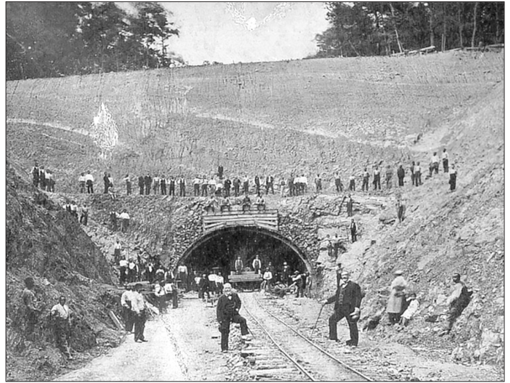
Andrew Carnegie (middle front) visits the Rays Hill Tunnel's eastern portal work site in Fulton County in 1880.
